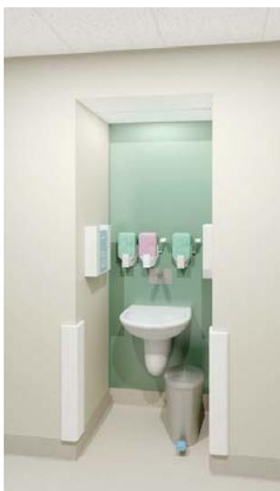
Figure 1.9: Reduced height ceiling within a corridor bay
