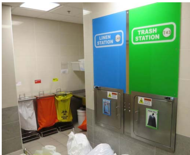
Figure 14: Linen and Waste chutes are not recommended
