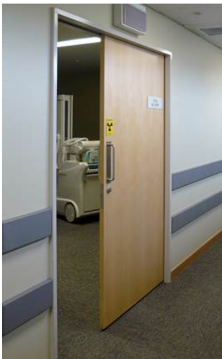
Figure 22: Cavity sliding doors not suitable for clinical areas
