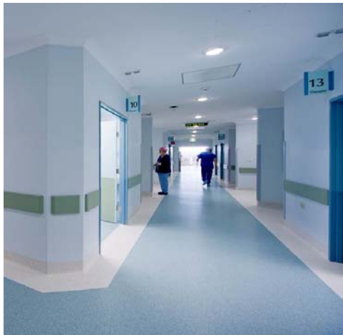
Figure 23: Floors and skirtings in clinical areas such as Operating Unit are integral and covered.
