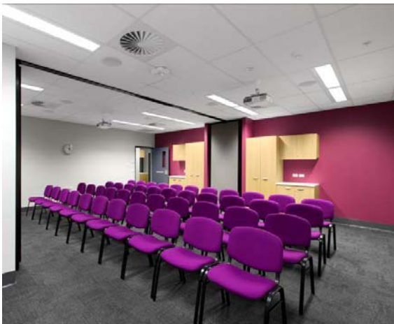
Figure 20: Acoustic tile ceiling suitable for offices, Conference rooms
