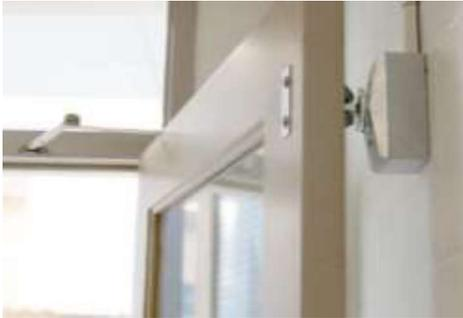
Figure 5.7: Electronic operated door hold open device
