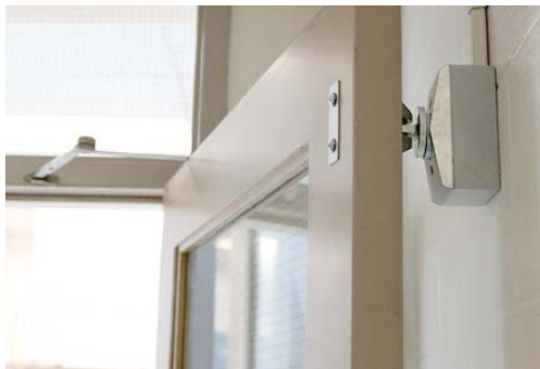
Figure 5.7: Electronic operated door hold open device
