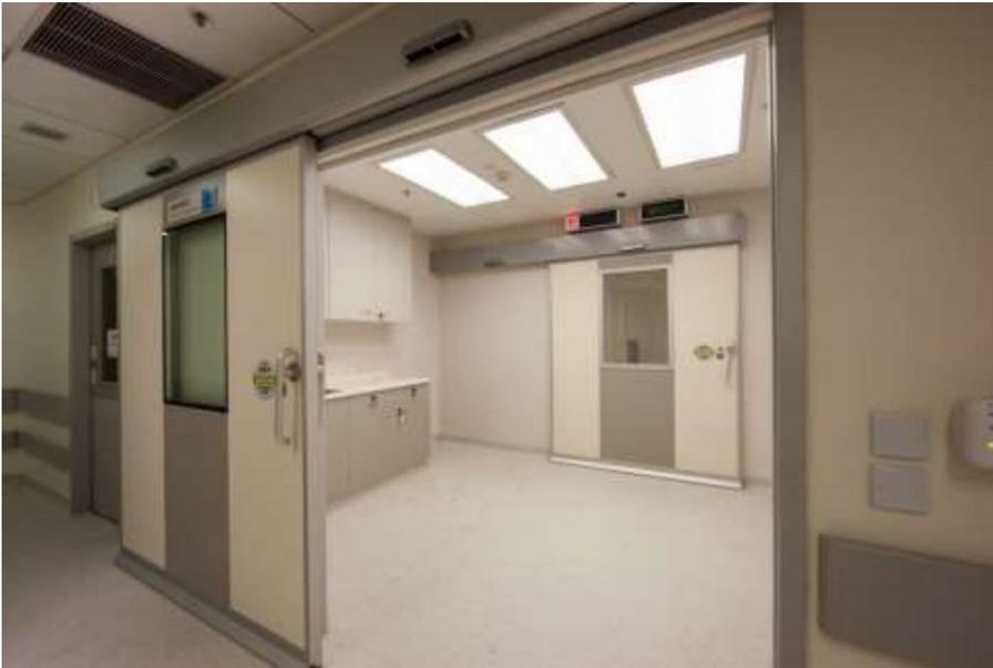
Figure 5.10: Surface mounted automatic sliding doors to Anaesthetic and Operating Rooms
