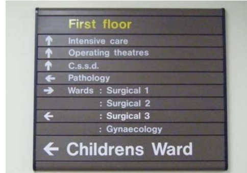
Figure 4.8: Removable slat type signs, with a locking cap
