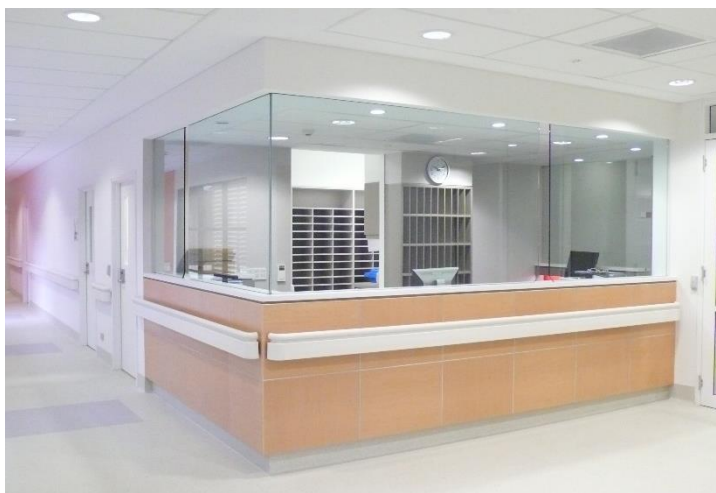
Figure 3.5: Staff Station with security glazing barrier
