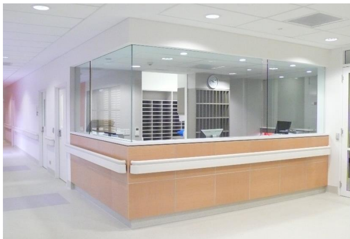
Figure 3.5: Staff Station with security glazing barrier used in a mental health facility
