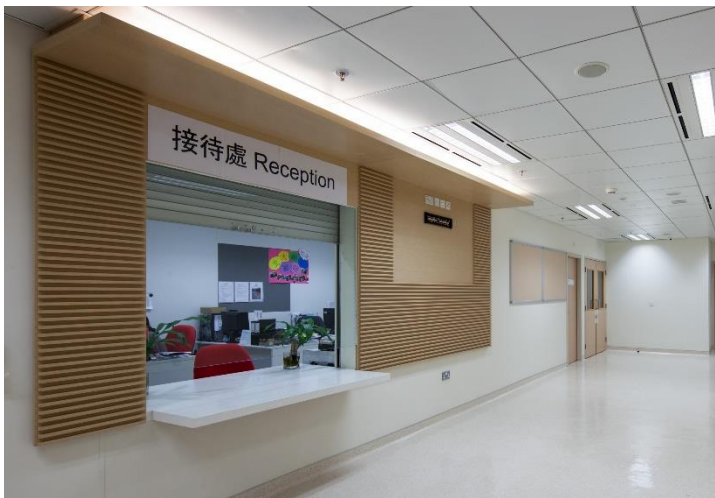
Figure 3.7: Reception with vertical roller shutter for after-hours security
