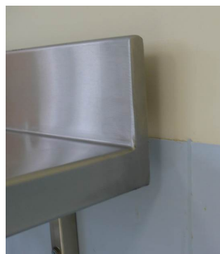
Gap between bench fitting and wall
