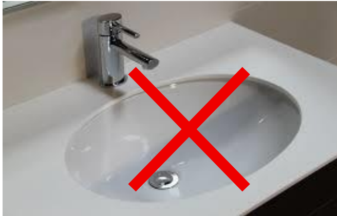
Figure 4: Under mount hand basin is not recommended
