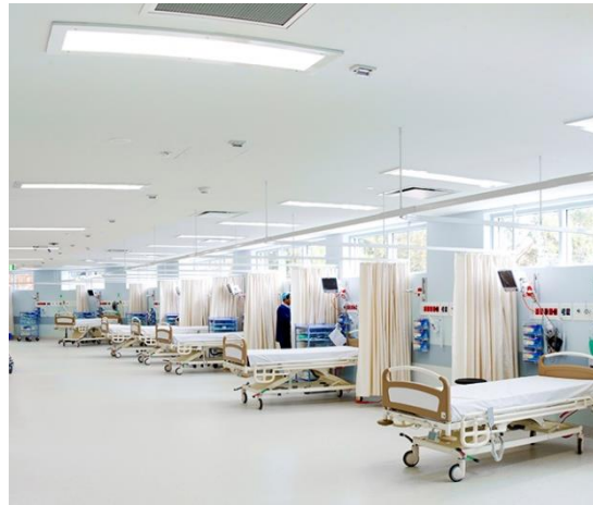
Figure 23: Monolithic ceilings in Stage 1 recovery areas
